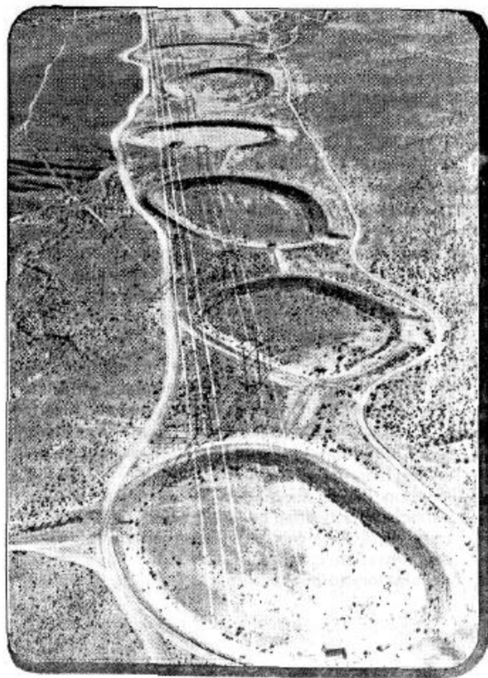
THE LADERA DETENTION DAMS, PNM CORRIDOR
