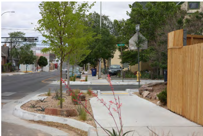
Bulbout improvement on Lead Avenue.
