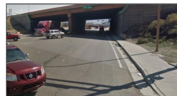
Comanche EB at I-25 Overpass - 2 lanes with no shoulder
