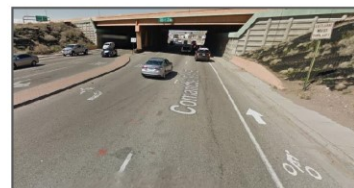
Comanche WB at I-25 underpass
